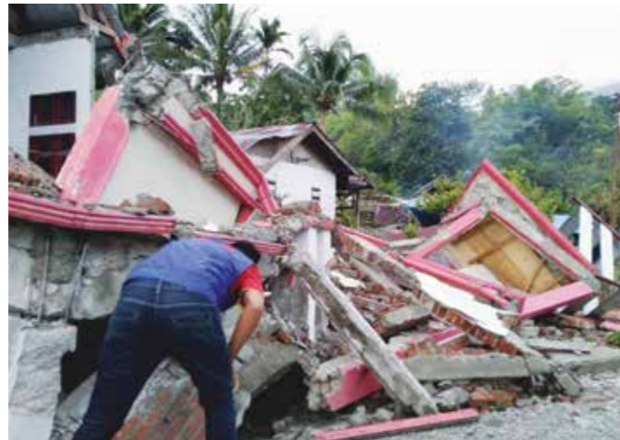
^ One of the many Salvation Army properties damaged during the earthquake and tsunami in Indonesia.
