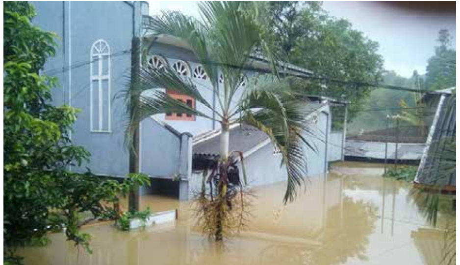
The Salvation Army church and community centre in Ratnapura, south-western Sri Lanka, experienced severe flooding and extensive damage.
