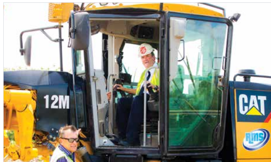
Commissioner James Condon climbed aboard some heavy machinery to symbolically 'break the ground' on the site of the new Northern Queensland Recovery Services centre.
