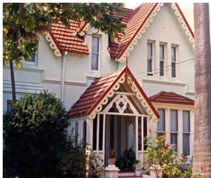
Front view of the refurbished Lodge.
